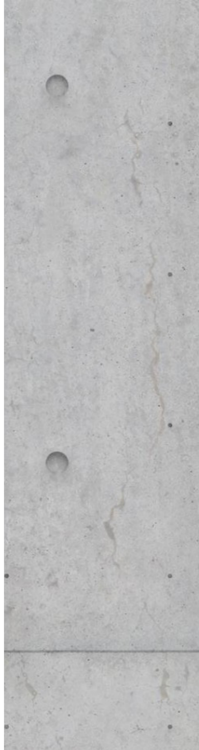
OFF-FORM IN-SITU CONCRETE
